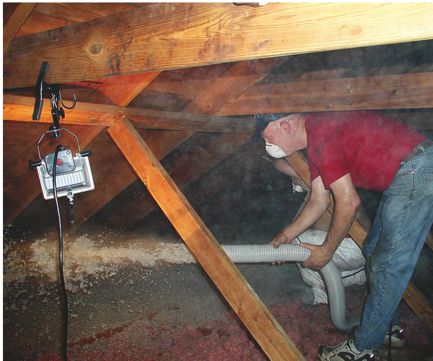
When blowing cellulose insulation into the attic, make it snug. "A few extra few bags of insulation just doesn't add that much to the cost," says Tony Karpovich of GreenHomes America.
