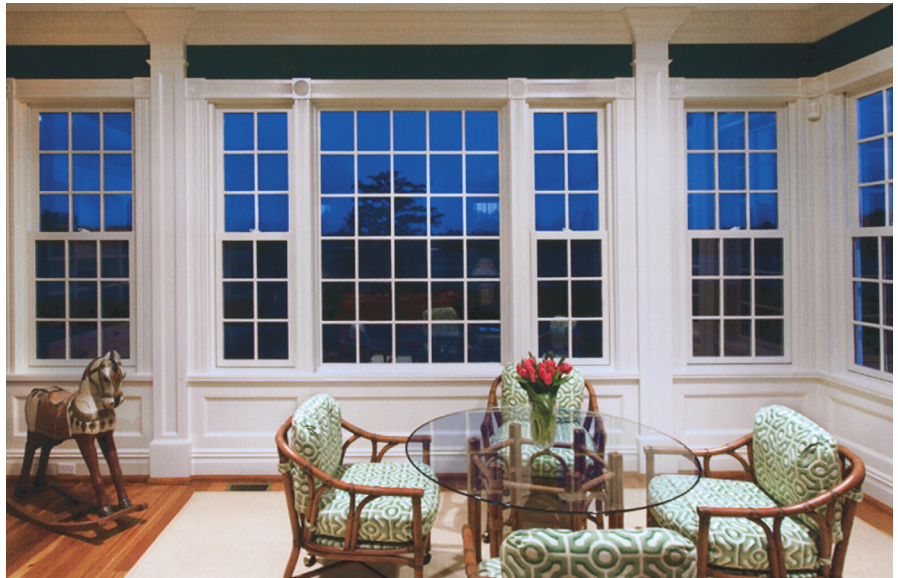
The sunroom features true divided light windows with real wood jambs that look like those found in an older home, but the insulated, high-performance glass is clad in aluminum, which creates an almost maintenance-free finish. "The addition needed to be sunny and provide a lot of views, and there was no room in the existing house that did either of those things," remodeler and architect C. Mason Hearn Jr. says. "But we still measured the window panes in the existing house and kept the ones in the addition similar to or equal in size."
